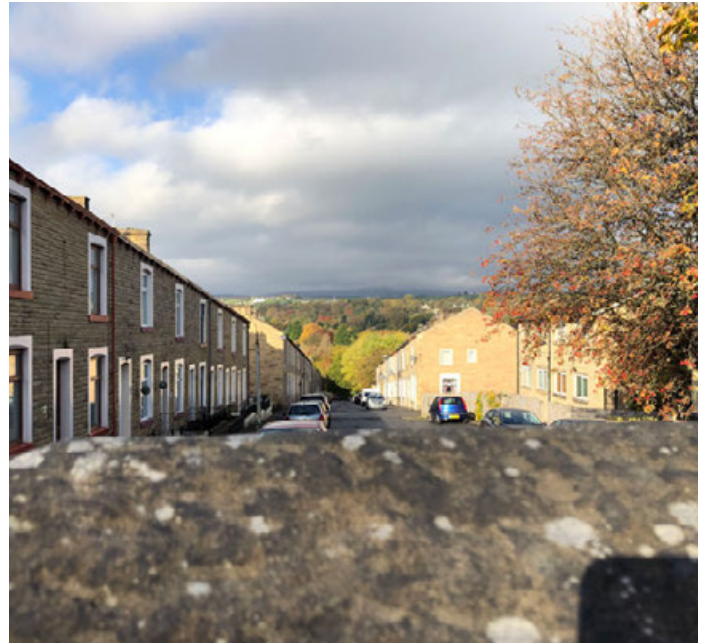
Enclosing walls in Nelson create access barriers and poor connections to the town centre with developments turning their backs to the canal (Pendle)
