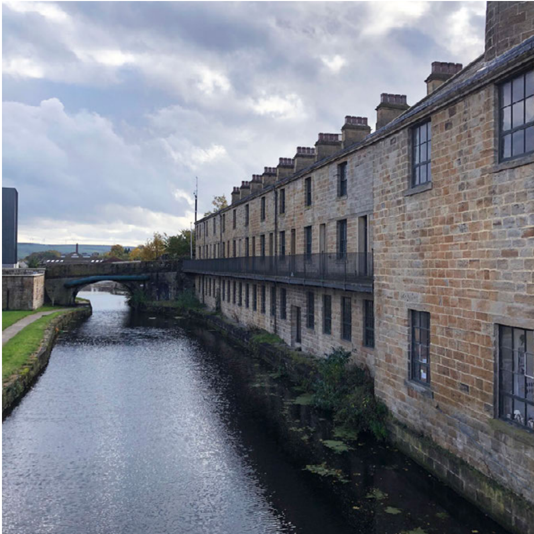
Weaver's Triangle has a sense of place defined by its sequence of mill buildings, weaving sheds and canal-related structures, some occupied with new businesses but many still vacant and in a state of dereliction (Burnley)
